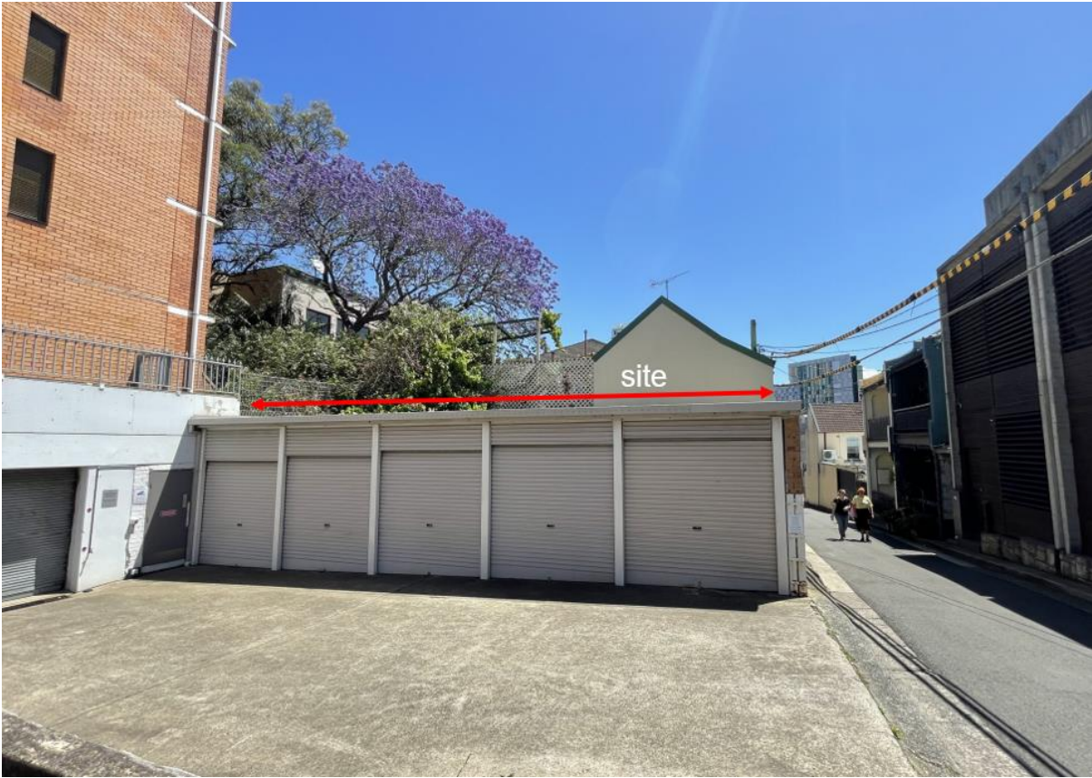
Figure 4: West elevation viewed from Wells Street
